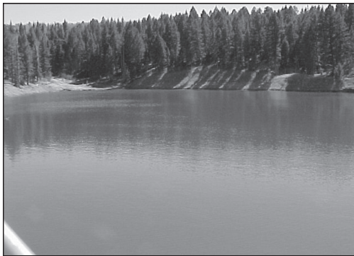
Woodland Park's Loy Gulch Reservoir provides for local storage of augmentation water imported from Twin Lakes near the Continental Divide.
