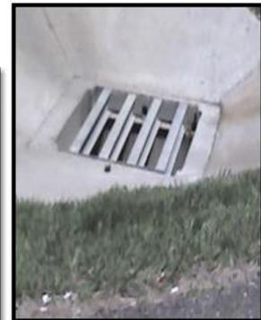
**Photograph 8-7.** CDOT Type C Grate Inlet (UDFCD Volume 1)
