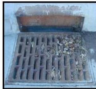
**Photograph 8-6.** Denver No. 16 Combination Inlet in need of maintenance (UDFCD Volume 1)
