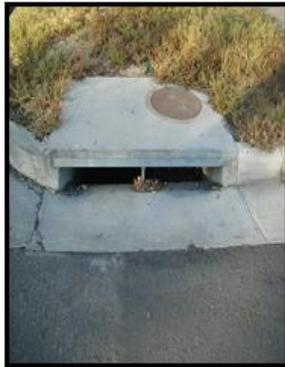
**Photograph 8-4.** Denver No. 14 Curb Opening Inlet (UDFCD Volume 1)
